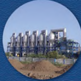
YEMEN ASFALT PLANT
